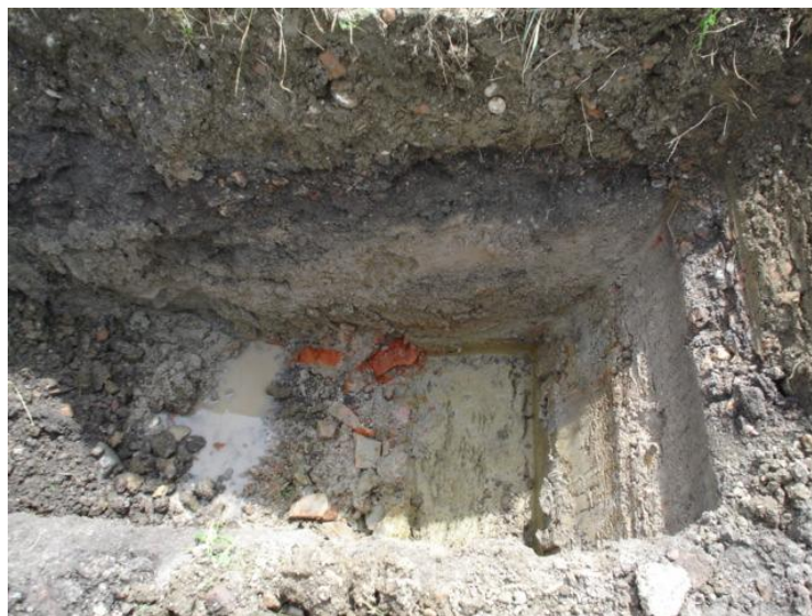
Fig. 17. The wall beneath the road.
