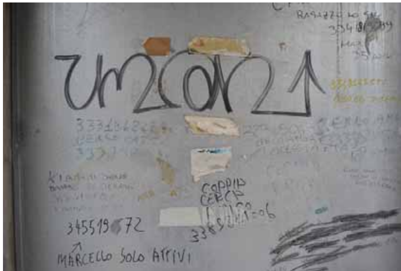
Fig. 8 A wall in the underground car parks. Now used as a board for private announcements.
