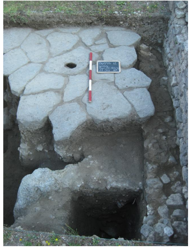
Fig. 22. Base of the opus incertum wall, at right, beneath the Phase 3 lava paving stones and wall (WF 1196/1198).
