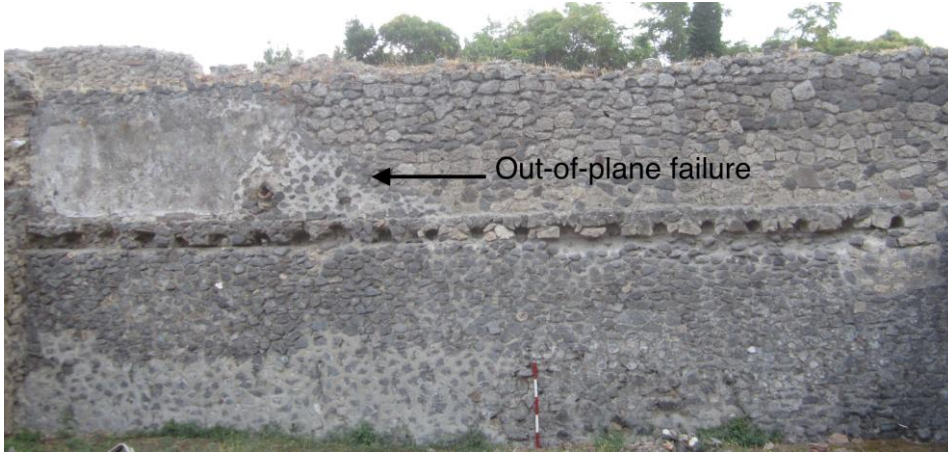
Fig. 17. The rear, easternmost wall (WF 1107) of property I.1.3-5; note the out-of-plane failure.
