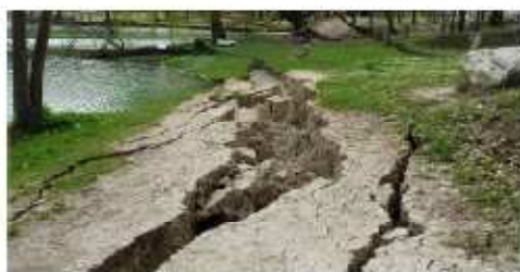
Fig. 9: Ground failures along the shore of Lake Sinizzo
