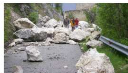
Fig. 8: Fossa rockfall: huge boulders on a paved road
