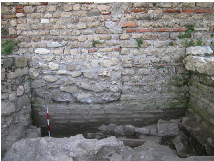
Fig. 18. The foundations of a Roman building under the blocked door of the church.
