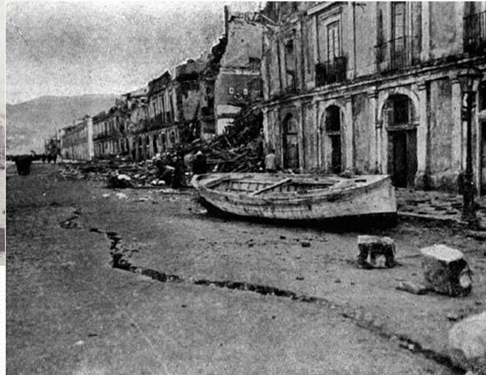
Ground crack along Marina Street, Reggio Calabria (Baratta 1910)
