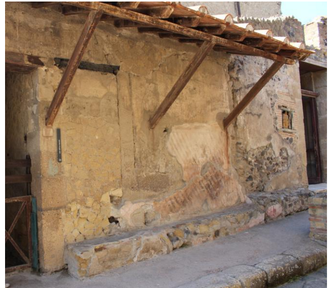
Fig. 7. Façade between III.16 and III.17, with short roof protecting façade and benches.
