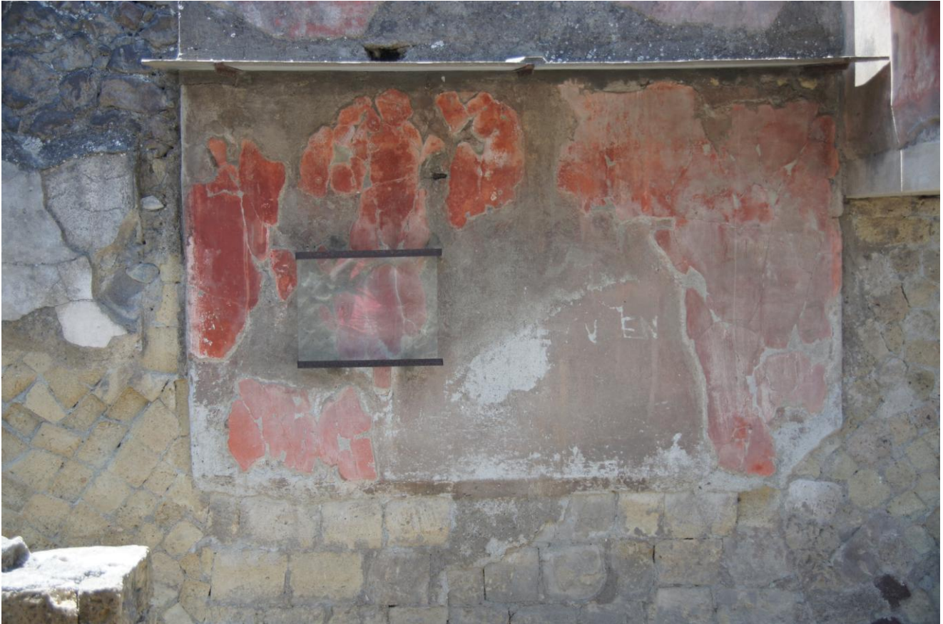
Fig. 10. Conservation measures have preserved CIL IV.10520 at the Casa del Papiro Dipinto (IV.8-9).
