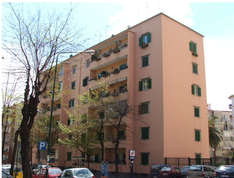
Fig. 6 One of the buildings of Rione Gemito
