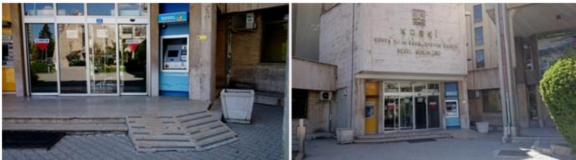
Fig. 4-c Building entrances in the survey area
