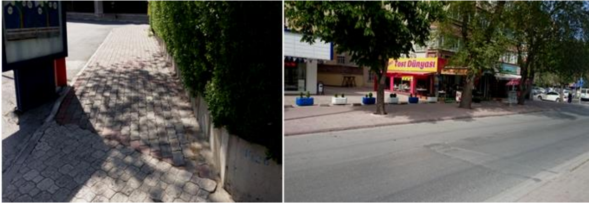
Fig. 6-a Pedestrian pavements in the survey area
