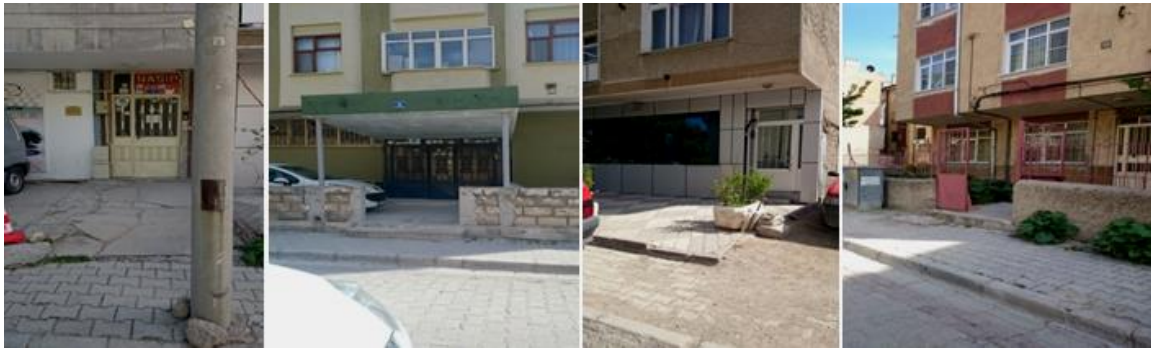
Fig. 4-a Building entrances in the survey area
