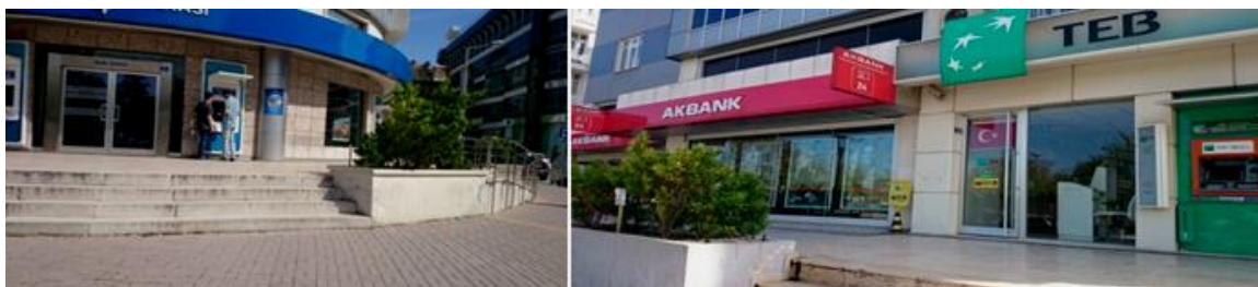
Fig. 4-e Building entrances in the survey area
