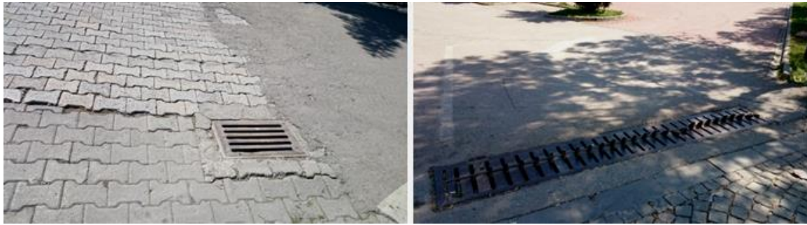
Fig. 7-c Technical substructure in the survey area
