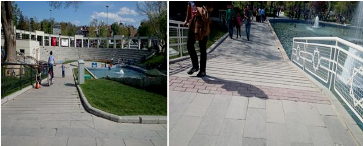
Fig. 7-a Ramps in the survey area
