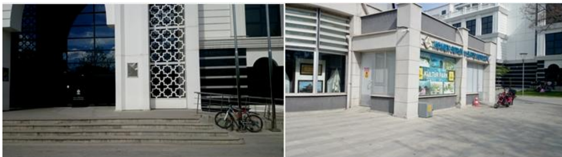
Fig. 4-d Building entrances in the survey area
