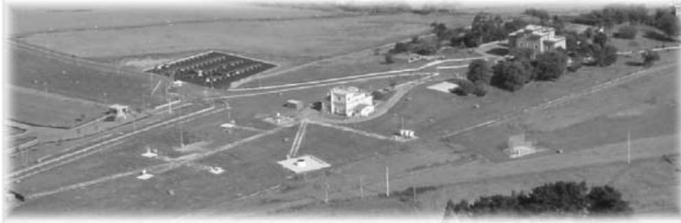
Fig. 4. – Aerial picture of ReSMA. The Experimental Site includes six equipped areas under both automatic and manual control everyday.
