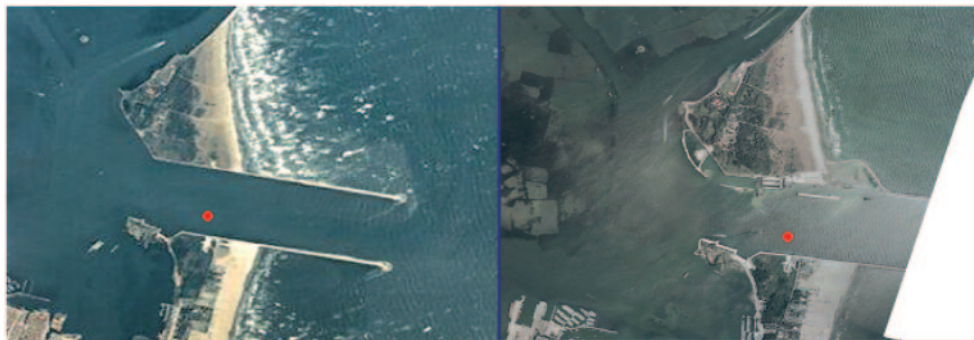
Fig. 2. – Aerial photograph of Chioggia inlet before (left) and during the construction works (right). Note different horizontal scales. The construction of fishery vessels’ haven is evident along the northern shore of the inlet in a more recent photograph. The position of the ADCP is presented by a dot.
