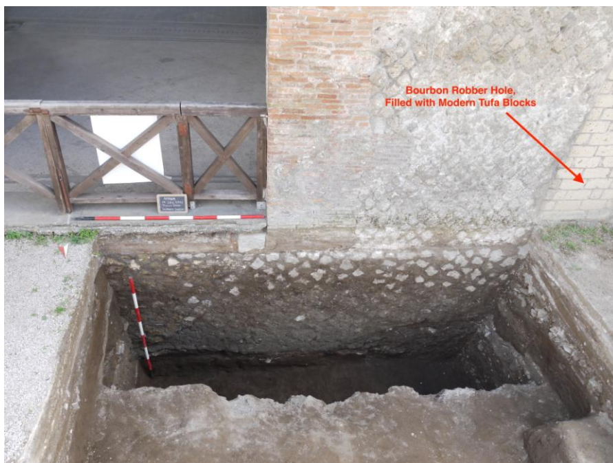
Fig. 12. Wall separating rooms 68 and 59. Foundation wall in opus incertum , wall in opus reticulatum , doorway in brick. The yellow tufa stones to the right are the modern fill of a Bourbon-era robber hole.
