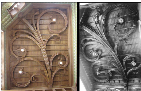
Fig. 2 – Two views of the final reconstruction of the ramage within Villino Florio.
