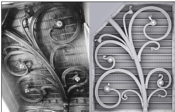
Fig. 1 – Comparison between the originale photo of the ramage before the arson (left), and the 3D reconstruction of the wooden ceiling (right).
