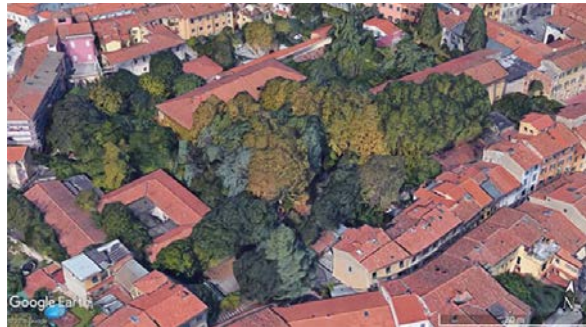
Fig. 3 The former Military District "Curtatone-Montanara"
