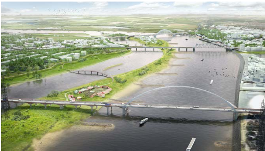
Fig. 4 - 5 Nijmegen. Room for the river project will create an island in the Waal and a unique urban river park
