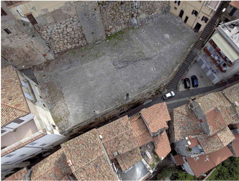
Fig. 4 – Piazza Pozzo Dorico substructures seen from above (photo by Giuseppe Guratti).
