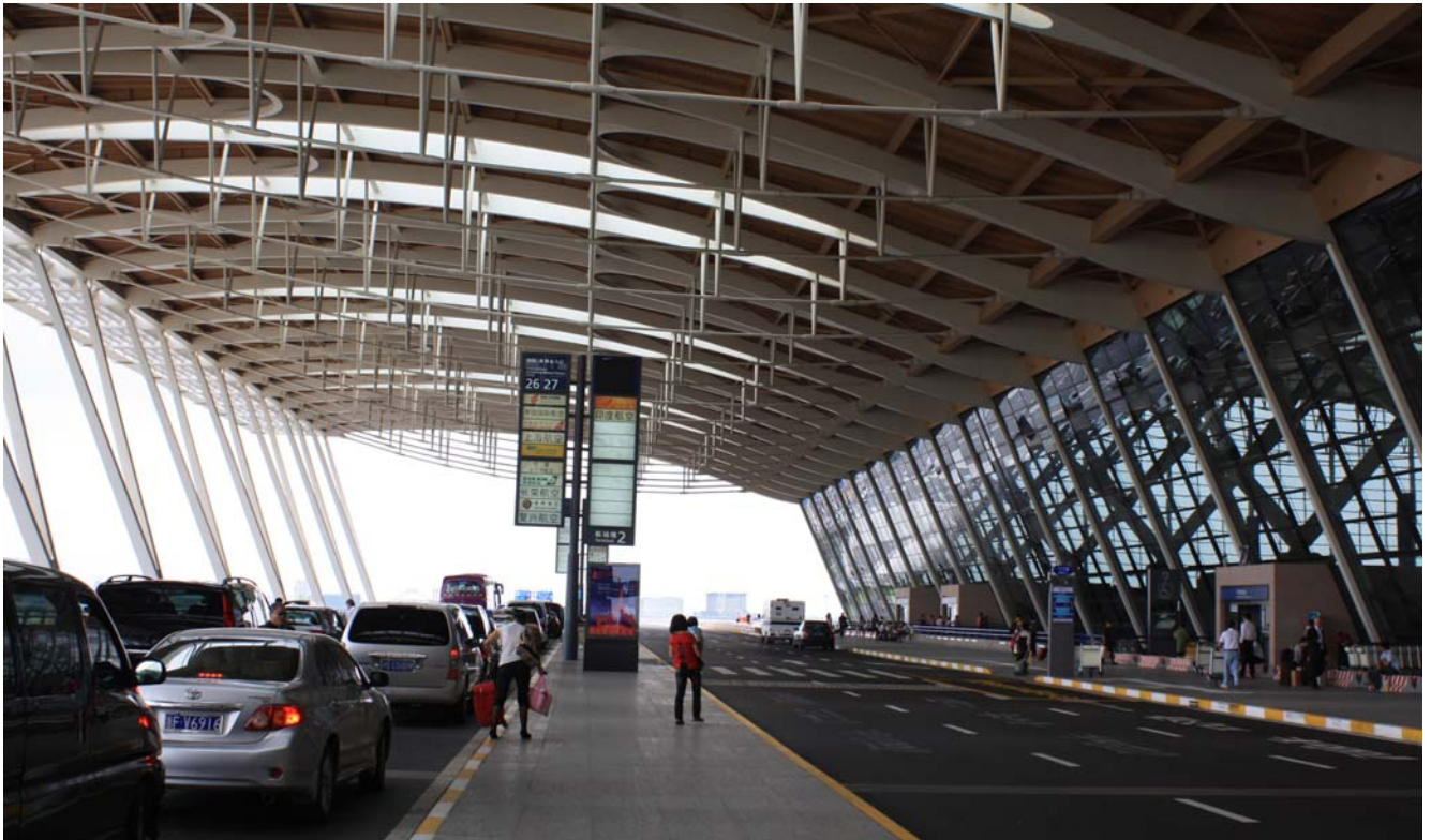
The external area of the Shanghai Airport with the covered six lane road for the car and bus arrival and departure of the passengers.
