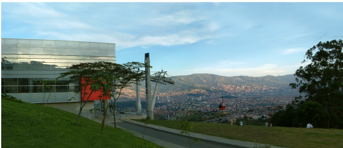
Fig. 9.- Terminal cable-car station of the West
