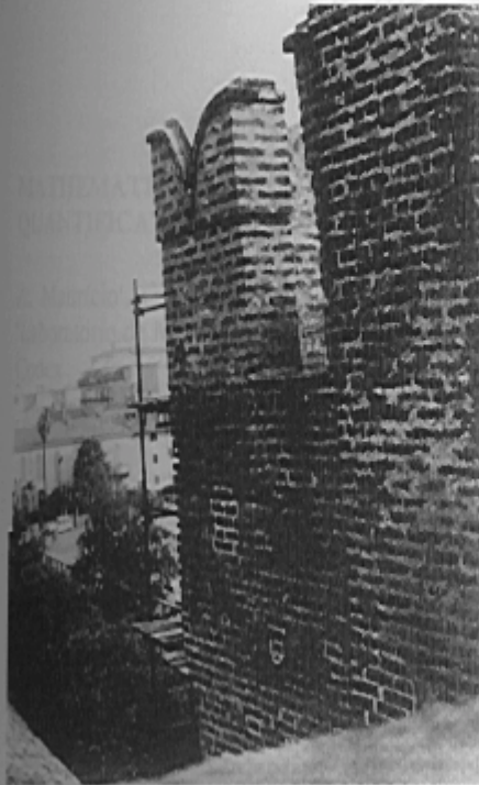
Fig. 1.1 - Crowing merlons of the south-east tower of the Sforza Castle in Galliate
