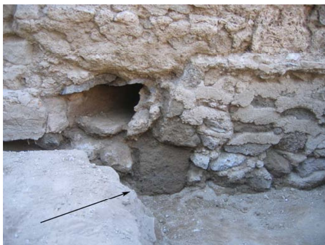
Fig. 4. Single pappamonte block below a later drain in WF 187 (looking north).
