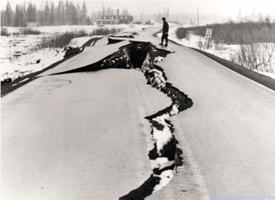
Damage to the Seward Highway caused by the 1964 Great Alaska Earthquake. Photograph by the U.S. Army.
